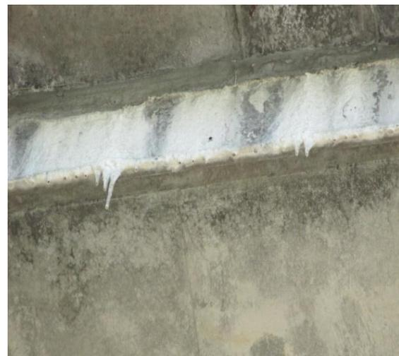
Fig. 6. Concrete leaching of over-bridge constructions
