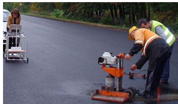
Fig. 9. Core sampling (right) while the received sensing data are processed (left)
